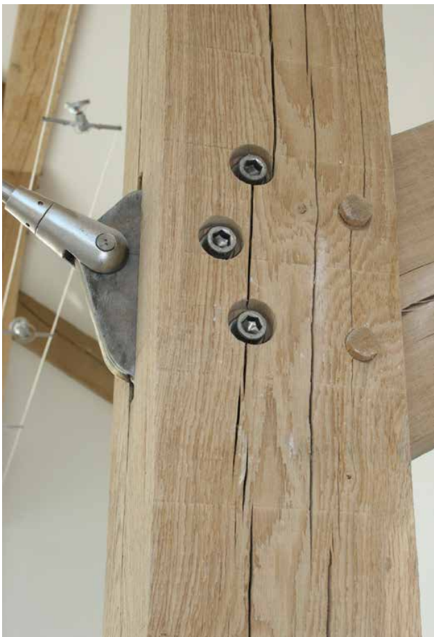
Figure 6: Modern metal joints in green oak Photo: Carpenter Oak and Woodland
