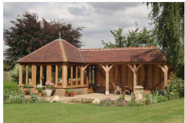
Figure 3: Green oak summerhouse Photo: English Heritage Buildings
