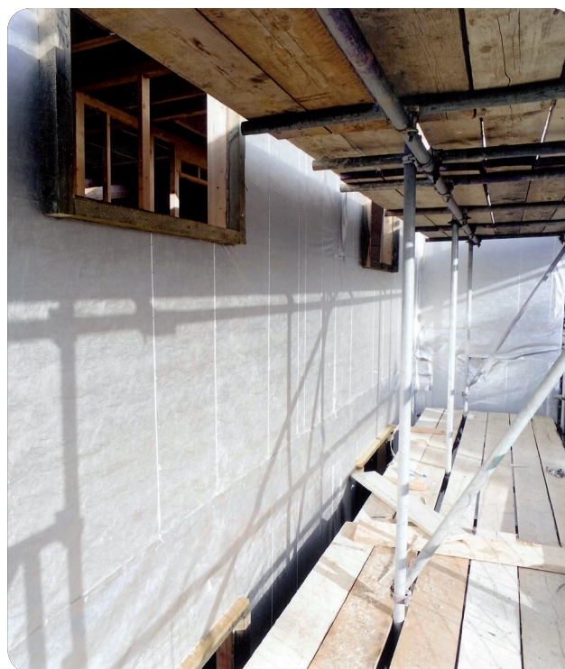
Figure 1: DuPont™ Tyvek® Reflex advanced breather membrane used in residential project in Burwell, UK.
