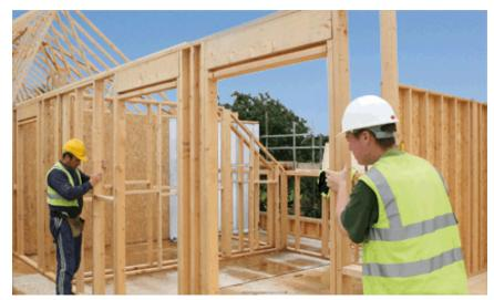
Figure 2: Installing open panels. Photo: Castleoak Group
