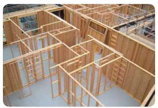
Figure 1: Modern timber frame construction
