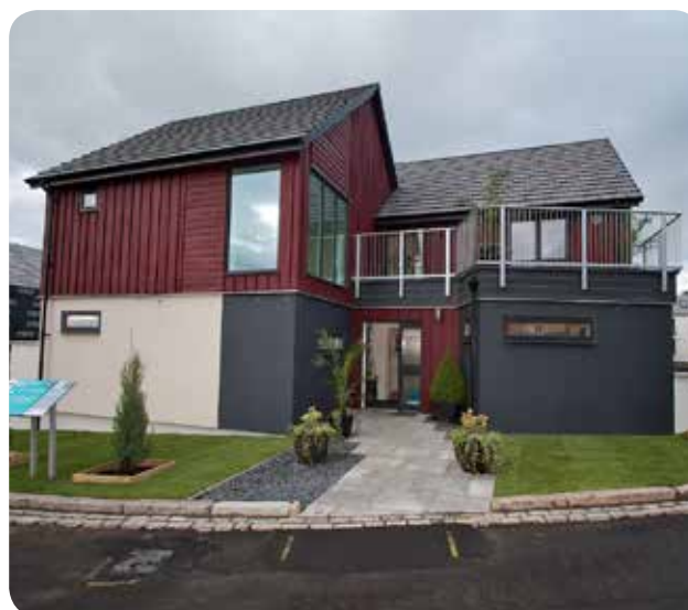
Figure 1: Timber frame house with a combination of vertical and horizontal timber cladding and rendered cladding
